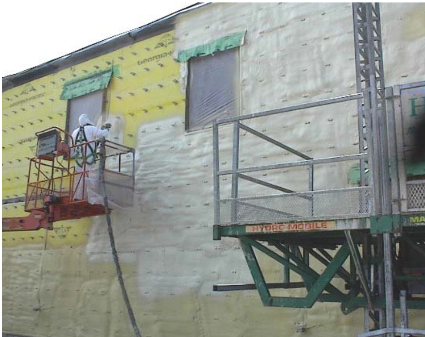
This picture shows the shell of the original building being insulated and air sealed. Construction began in 2005 and ended in 2008. The school has already seen significant energy savings.
