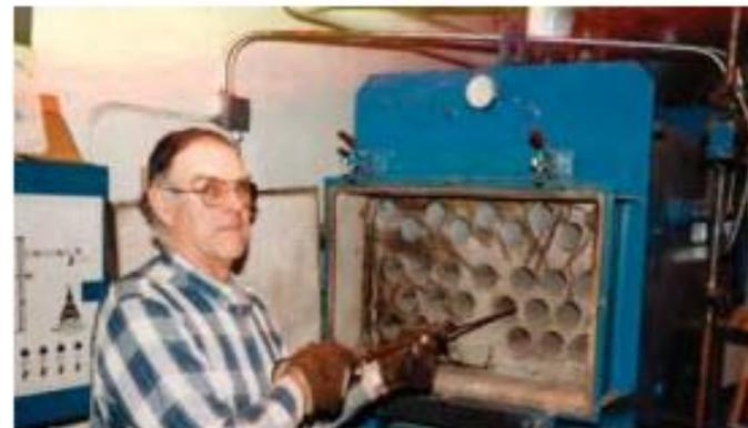
*Manual boiler tube cleaning at Calais Elementary School, Calais, Vermont (from the Biomass Energy Resource Center's Wood Chip Heating Systems)*
