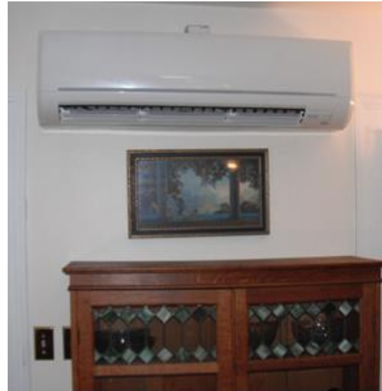
Figure 3: A ductless heat pump fan coil
