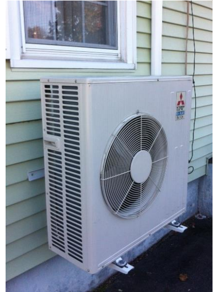
Figure 13: Cold-climate ASHPs operate at low temperatures, so it is important to keep outdoor units elevated and unobstructed from snow and ice. (Photo credit: Joe Swift)
