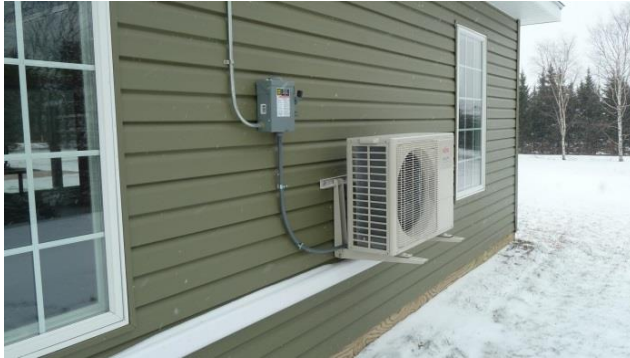
Figure 16: An inverter-driven ASHP in a snowy climate.
